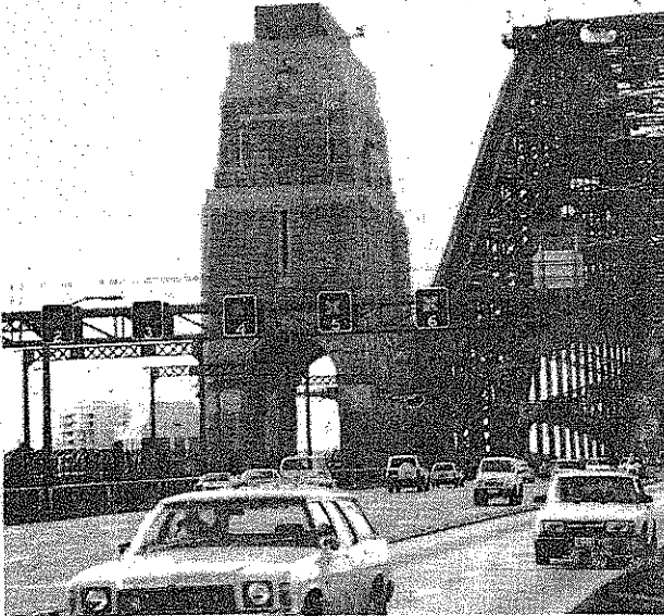
Figure 6.4.4 Contraflow operations are common on many busy bridges worldwide. Sydney's Harbor Bridge is pictured. (Photograph by P. D. Prevedouros.)
