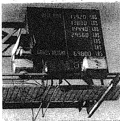
Figure 6.5.4 Weights per axle derived in Minnesota's Guidestar ITS program.
